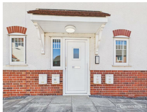
Communal entrance door with intercom entry system.
